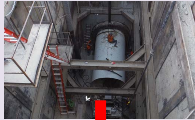
Conveyance to Central Basin (LADWP)
